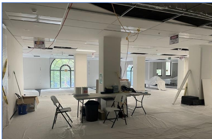
Photo 2 Mid-construction, looking from our (now open-plan) entry foyer towards Martin Place
